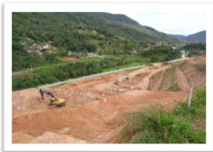
Florianópolis beltway (Litoral Sul toll road)
