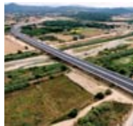
The work consisted of an extension to the motorway of 4.4 kilometres.
