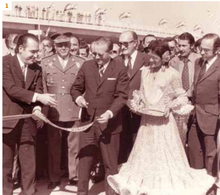
—1— On the 4th of November 1971, several sections of the road were opened: Dos Hermanas-Los Palacios; Los Palacios-Las Cabezas and Jerez South-Puerto Real. A couple of months later, the road was completed when the Las Cabezas-Jerez North Jerez North -Jerez South sections were opened.
