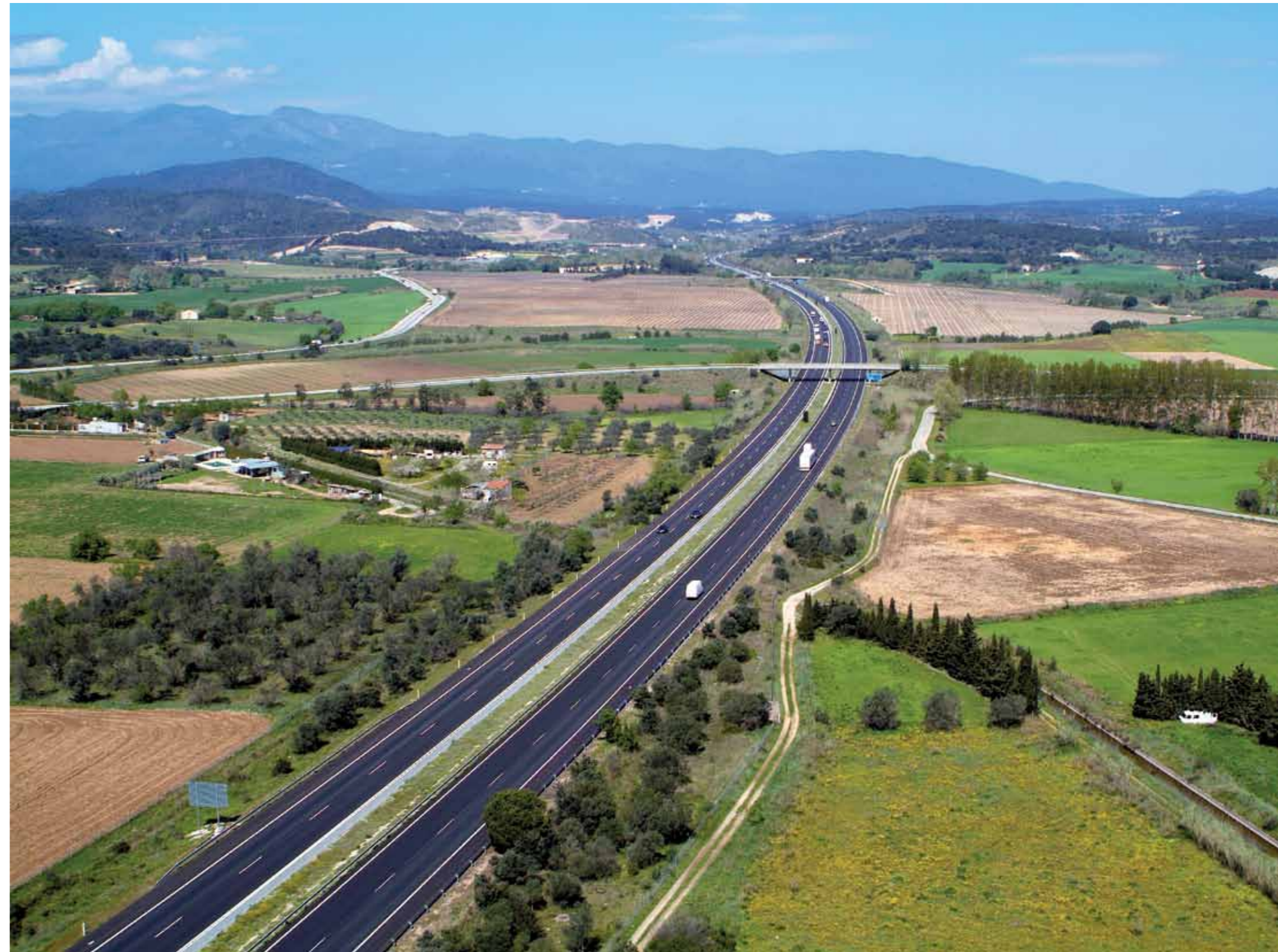
Aerial view of kilometre 18 of the AP-7.
