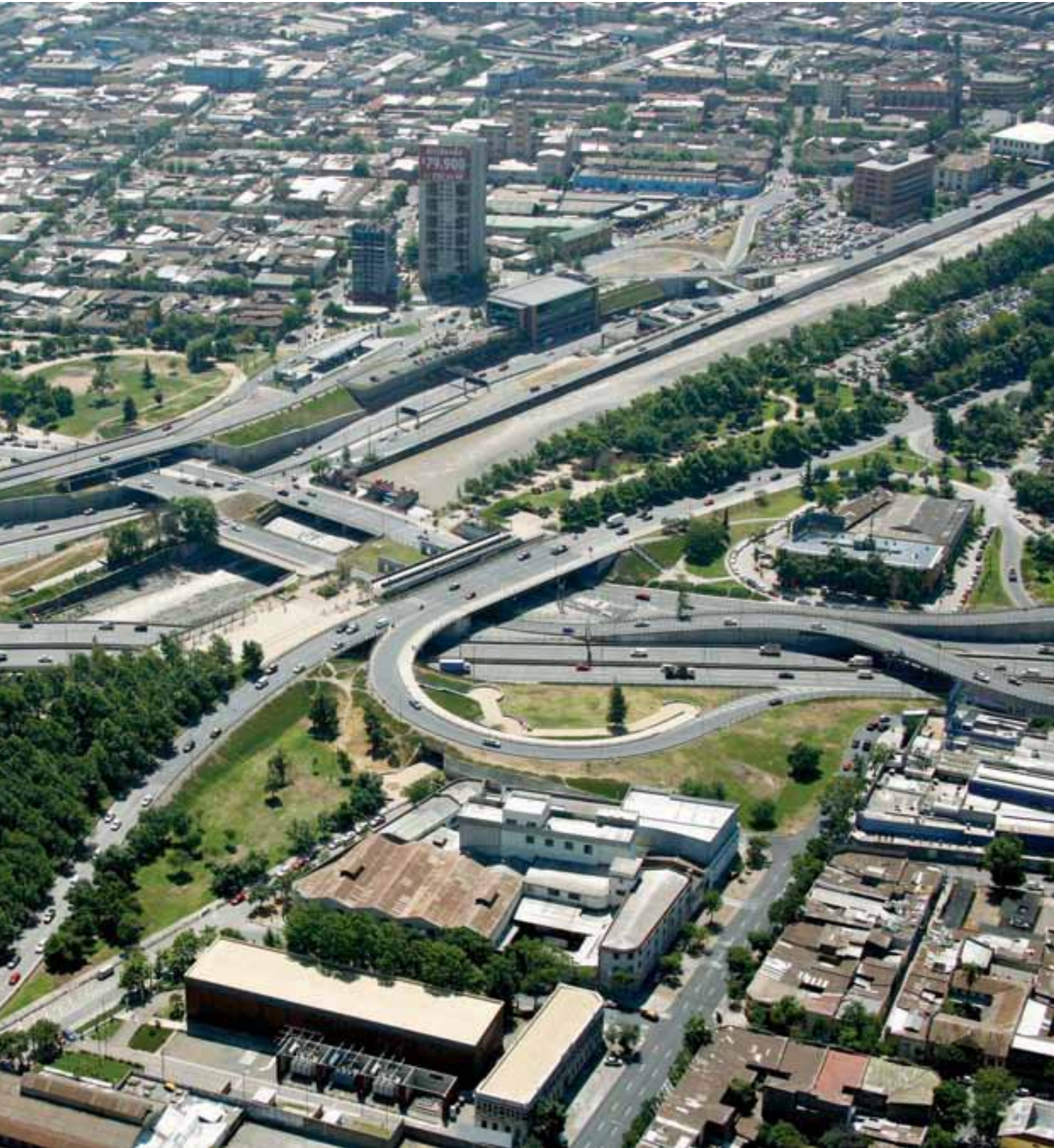
Section of the Vivaceta toll road, on the Autopista Central
