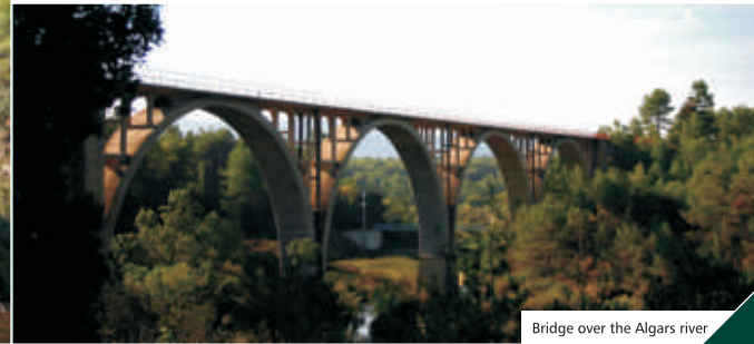
Bridge over the Algars river
